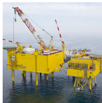
Dolwin Gamma HVDC Platform during the installation of the topsides
