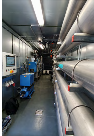
A new ultrafiltration plant for process water treatment reduces the water consumption and the malthouse waste water
