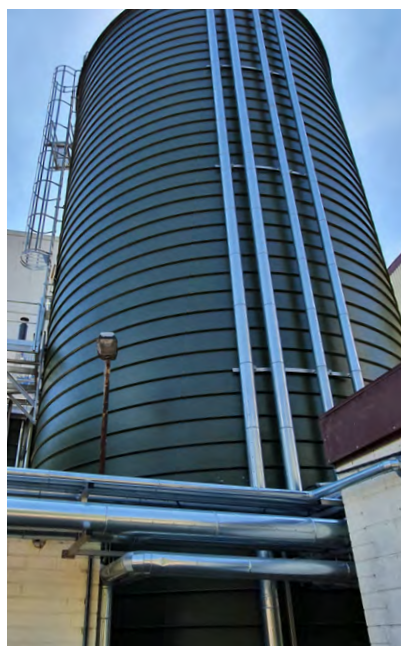
The process water tank has a capacity of 750 m 3
