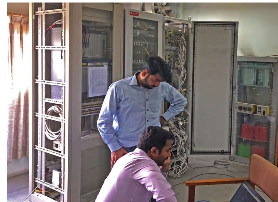
Point-to-point testing is used to check whether the SCADA system is working properly.
