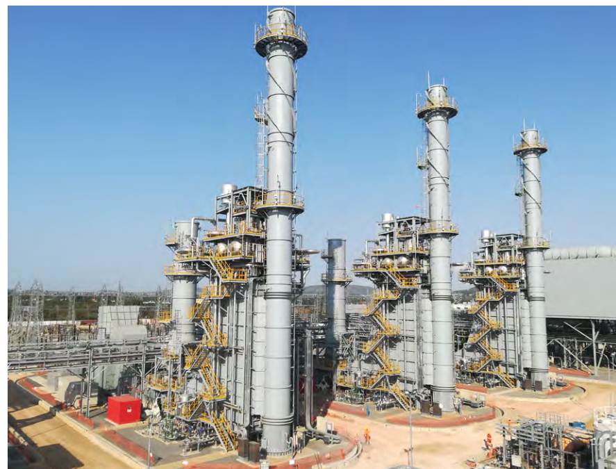
One of the two units with three gas turbines and three heat recovery steam generators.
