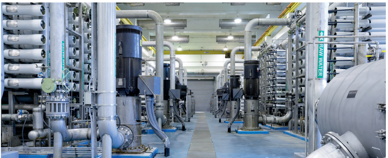
Inside a reverse osmosis desalination plant.
