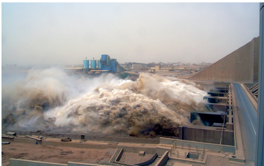
Flushing operation during flood season to prevent depositions in the reservoir
