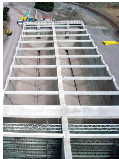
Desander with an integrated flushing device. Project: La Higuera HPP in the Chilean Andes.
