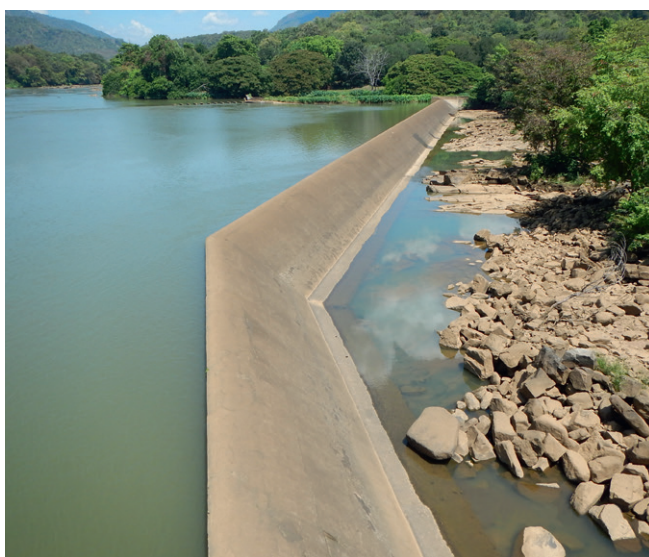
Irrigation diversion weir on the Mahaweli River, Sri Lanka
