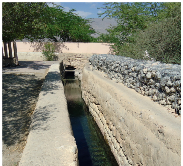
Water abstraction for agricultural use through Aflaj irrigation system, Oman
