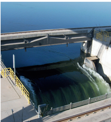
Naga Hammadi Barrage, Egypt: radial gate flap open
