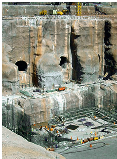
Rock excavation & foundation preparation for a surface powerhouse (Nam Theun II, Lao PDR)
